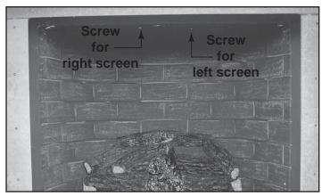
Figure 8.12 Remove Screws from Firebox Top
